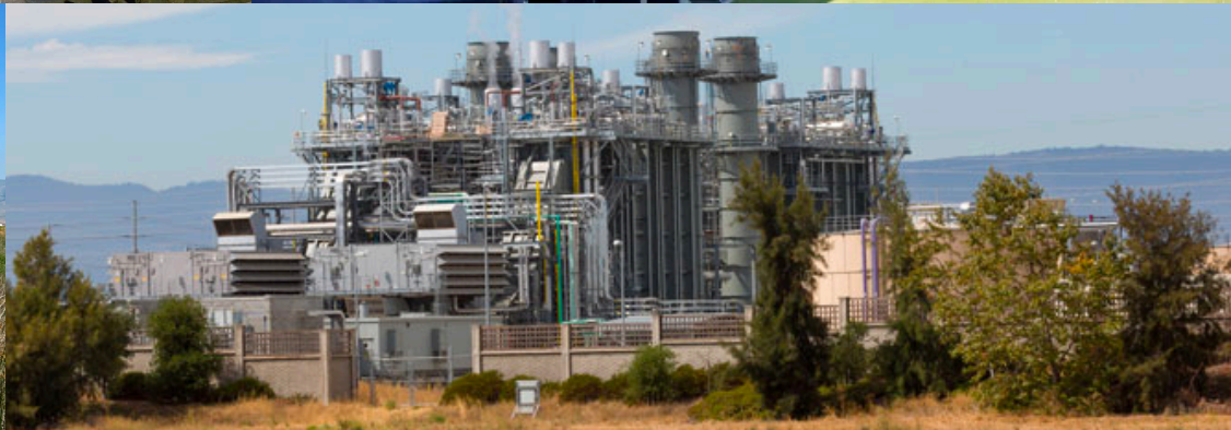
Calpine Los Esteros Energy Facility
